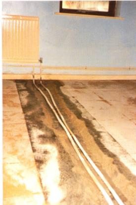
Leakage from pipes buried in the floor can result in considerable damage; disruption to locate the fault may be extensive, Figure 1.
