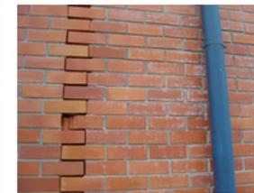
Cracking and splitting of the masonry wall near the expansion joint due to its inadequate width and significant irreversible expansion of fired clay brick
