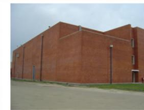
Typical facing brick masonry walls where expansion joints are required and where irreversible expansion of fired clay brick is a real risk
